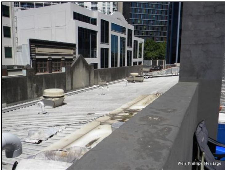
Figure 41: Nos. 761-763 George St – roof.
