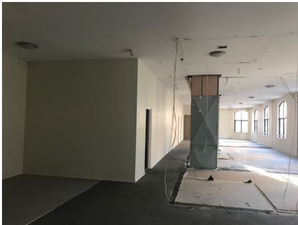
Figure 44: Nos. 761-763 George St First Floor interior.
