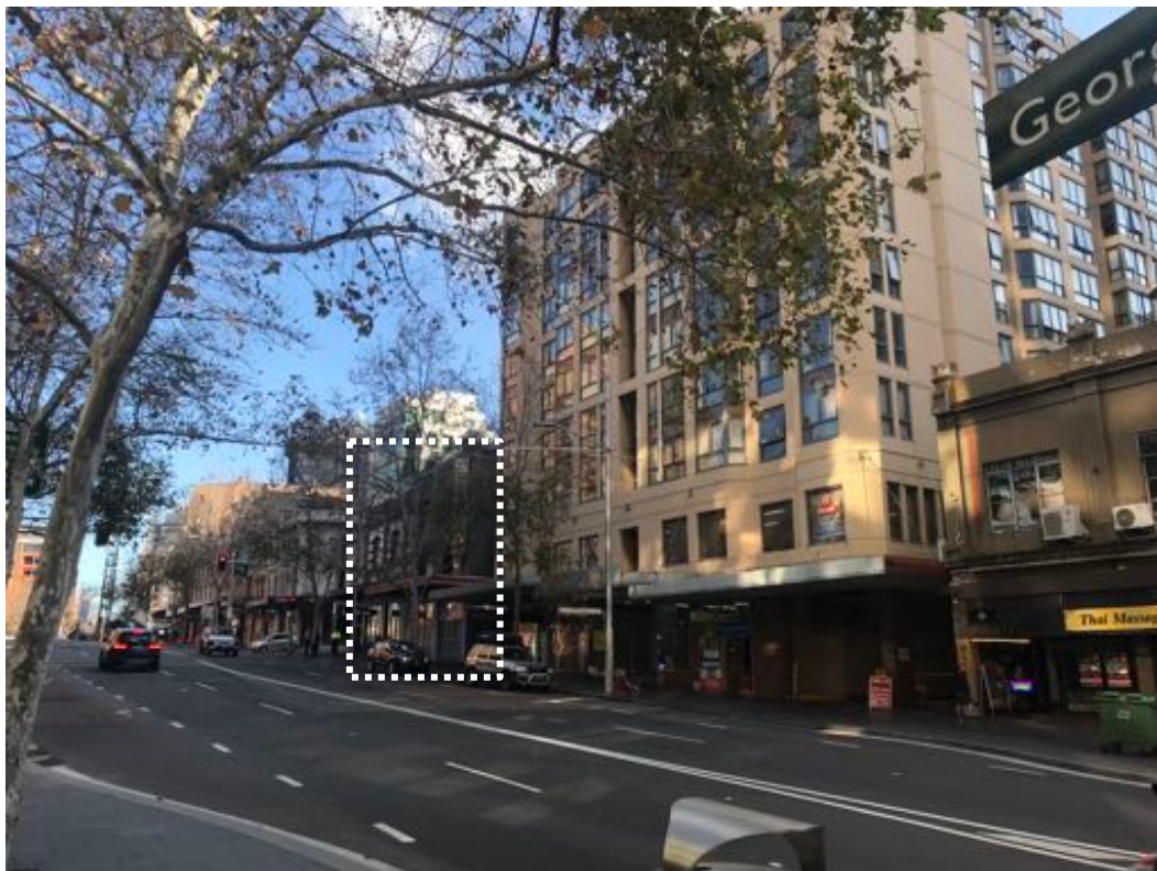
Figure 26: The site outlined in white, viewed from George Street looking south. Site outline in white.
