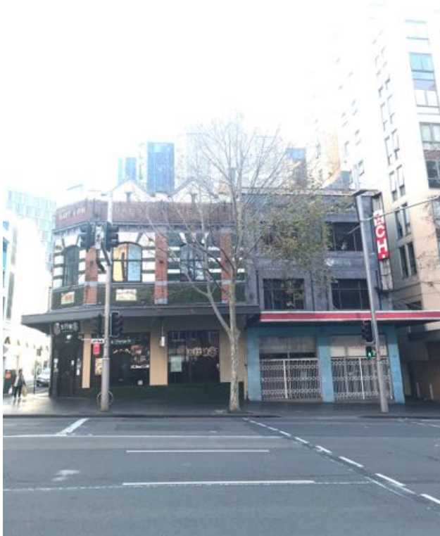
Figure 48: Nos. 757-759 George Street. From George Street.
